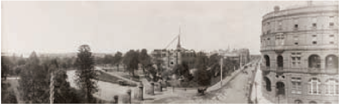
Photograph of Mitchell Library in course of construction, March 1907, ML V1/ Lib/Mit/2
